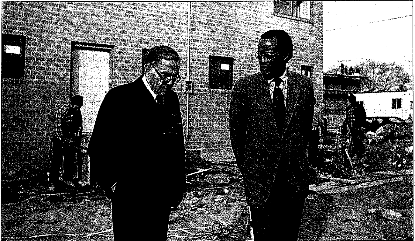
Williams and I.D. Robbins, founder of the Nehemiah Trust, survey the construction of low-income housing
